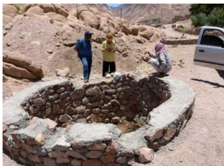
2 – The well & flood protection wall.
